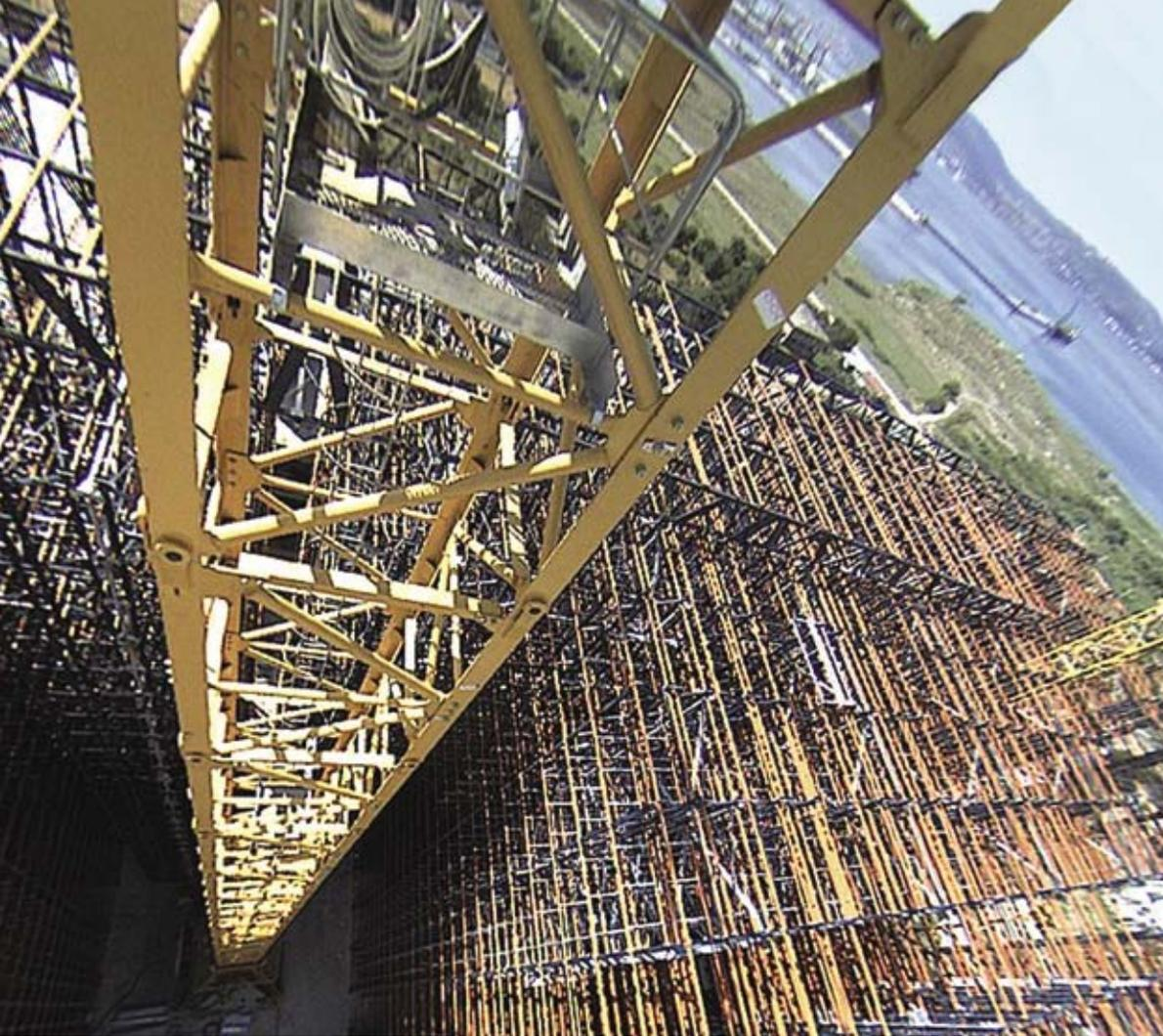
*AUTO HAYAT: As the 120-person work crew approaches the halfway point in the construction of one of the largest logistical facilities in the world, parallel to the assembly and mounting of the rack frames, the AS/RS units are beginning to be installed.*
