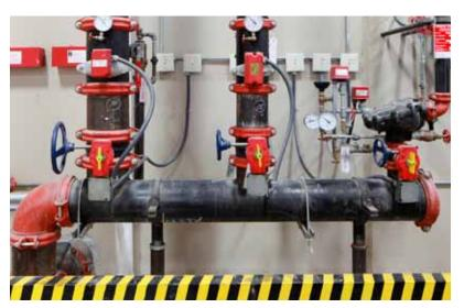
Valves for the industry's most common fire suppression system, the wet pipe.
