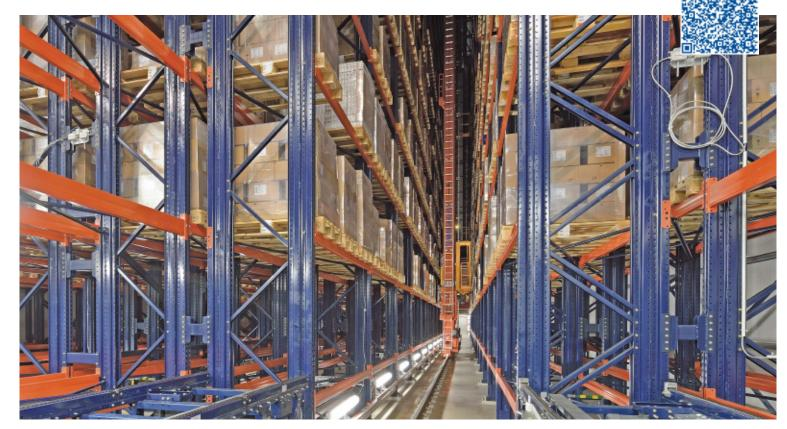
The solution was to construct a temperature controlled, 107' high clad-rack warehouse with a capacity to store more than 6,500 pallets. It is equipped with a cold storage system and an 'oxygen reduction system' for fire prevention. They were also supplied with a warehouse management system, the Mecalux Easy WMS, which is responsible for managing all the center's processes.
