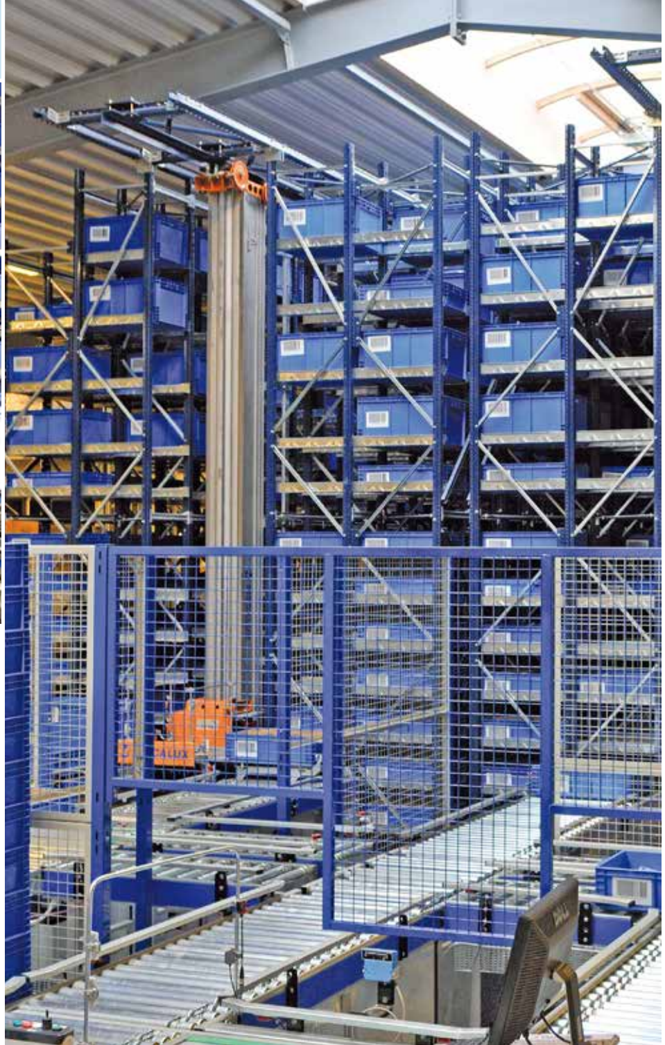
Warehouse with double depth
