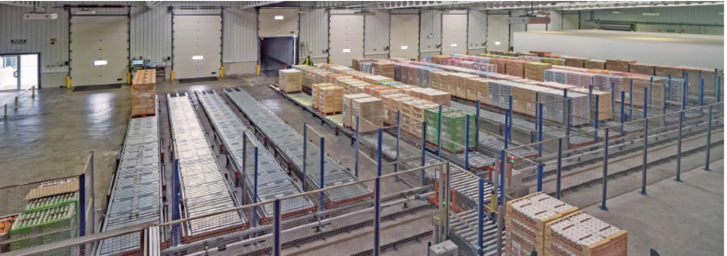
Pallets flowing from the warehouse or picking zones are sorted into preload channels using a transfer car.
