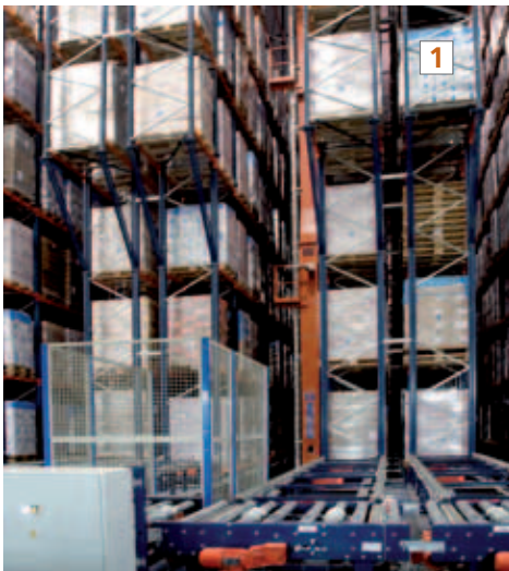
More products can be stored in the automatic conveyor rotation.
