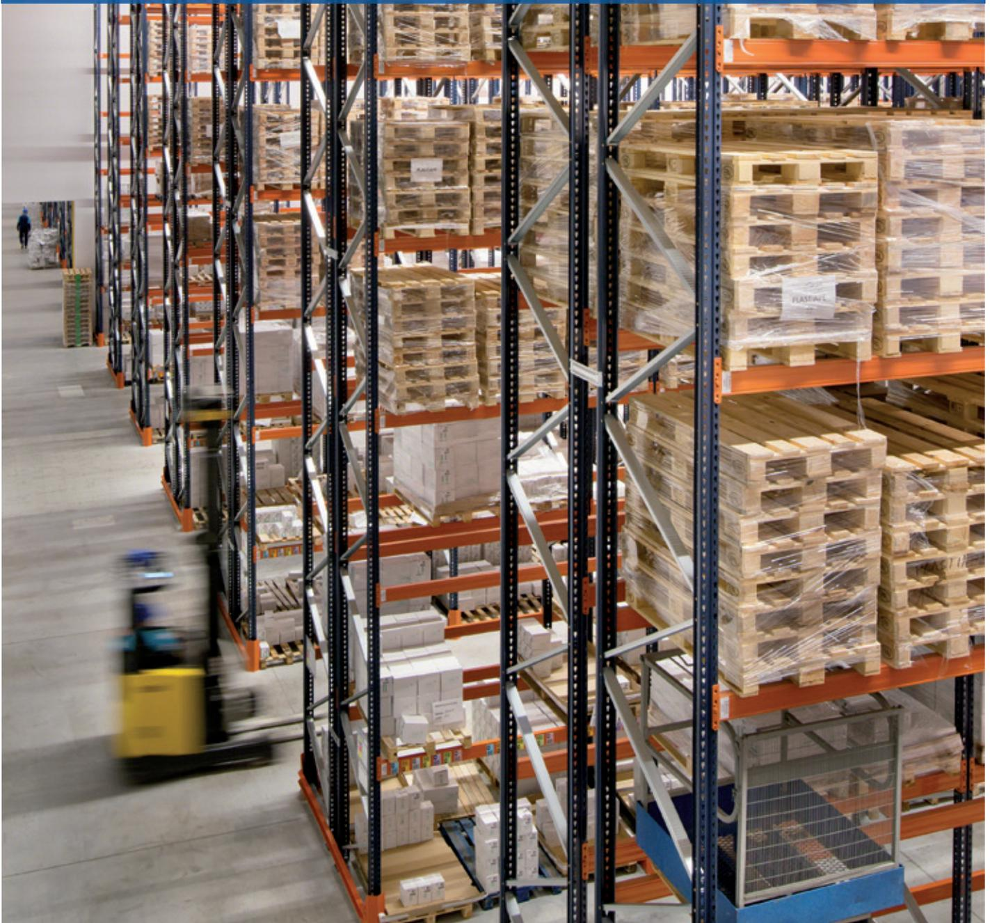
Ziaja, Polish manufacturer of natural cosmetics and pharmaceuticals, has a new warehouse designed specifically to streamline picking, the chief operation of the center. Mecalux has installed standard pallet racking, which offers direct access to the goods and has a storage capacity of 10,906 pallets.
