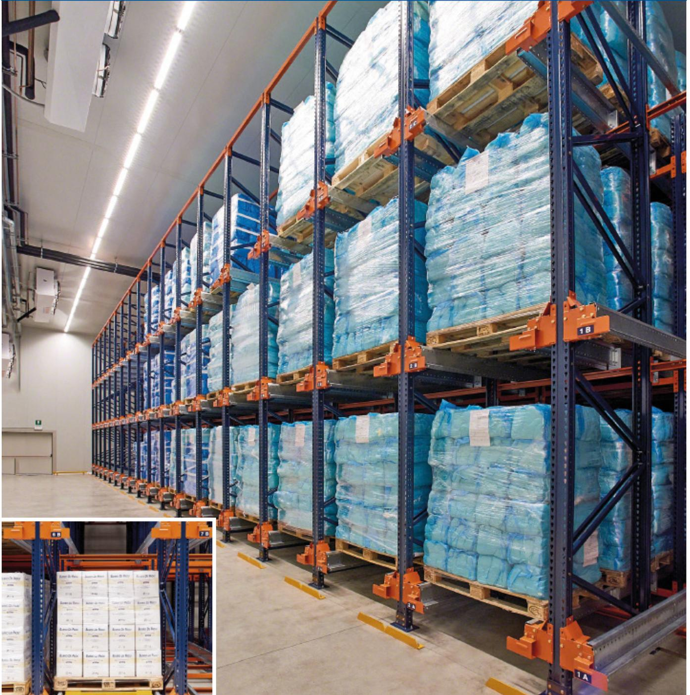
The butter producer Burro De Paoli has equipped both its frozen storage chambers in Italy with the semi-automatic Pallet Shuttle system. The installed storage solution boosts productivity, provides a 1,494 pallet capacity and minimizes the workforce.
