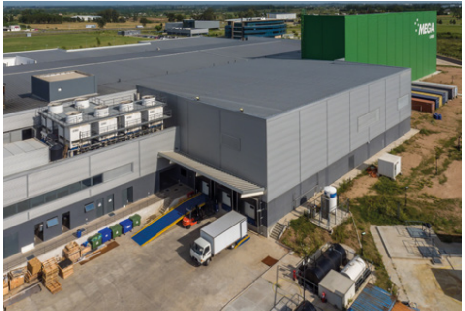
The loading and unloading docks are set off on their own to avoid interference between the two operations
