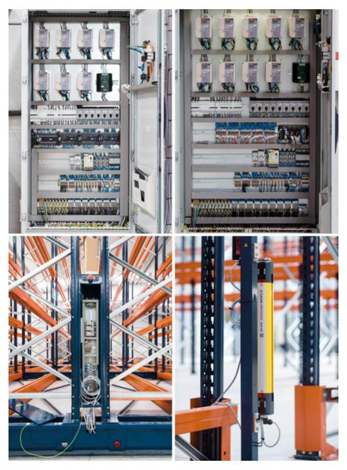
The Movirack units incorporate safety devices, such as external and internal barriers with photocells, which stop all activity when operators work inside the aisle
