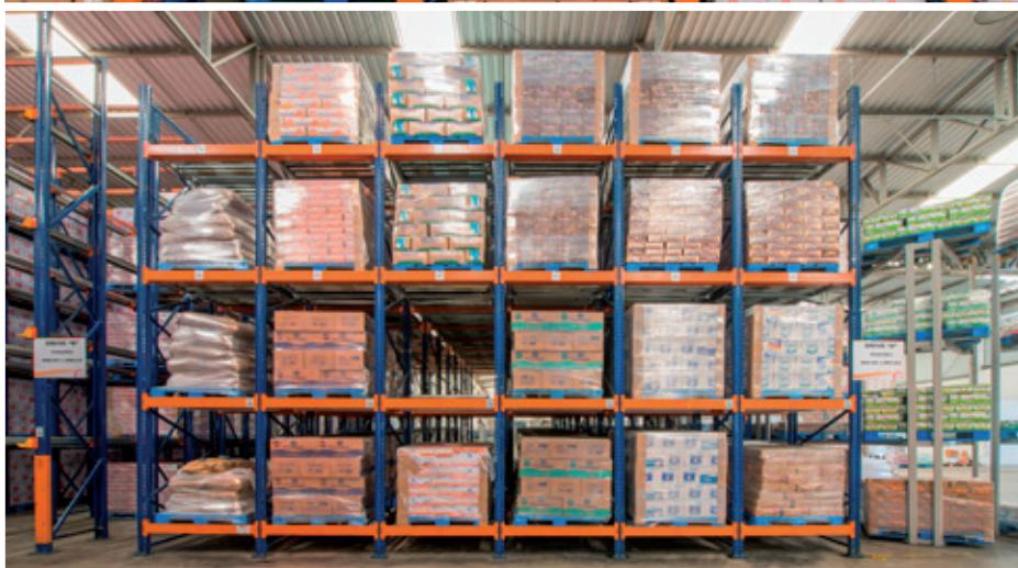
The Lacticínios Bela Vista company has purchased three different storage systems from Mecalux for its distribution center in Minas Gerais (Brazil): drive-in pallet racking, selective pallet racking and pallet flow racks. The installation has a storage capacity of 6,320 pallets, the best fit to meet the expected growth.
