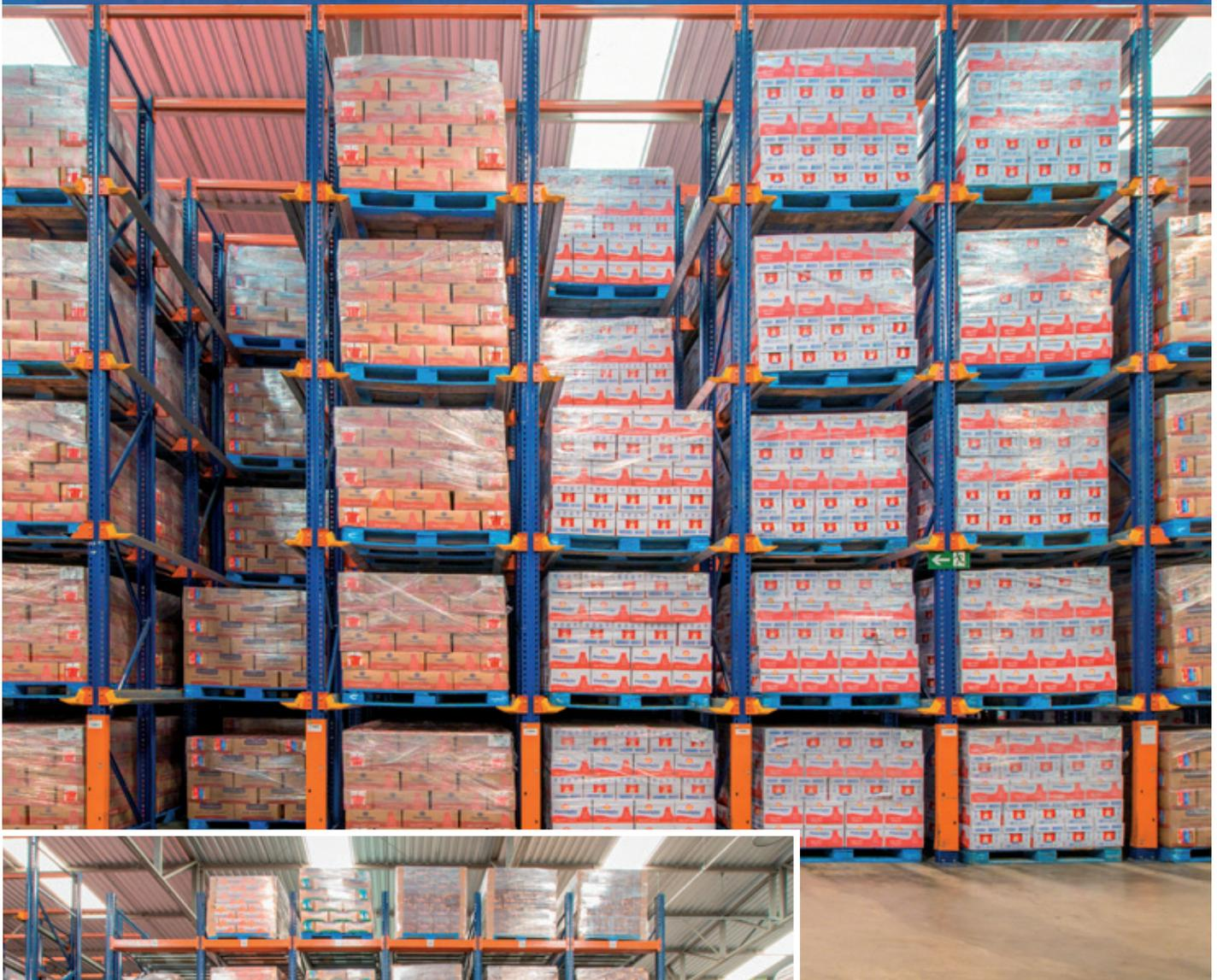
The Lactícnios Bela Vista company has purchased three different storage systems from Mecalux for its distribution center in Minas Gerais (Brazil): drive-in pallet racking, selective pallet racking and pallet flow racks. The installation has a storage capacity of 6,320 pallets, the best fit to meet the expected growth.
