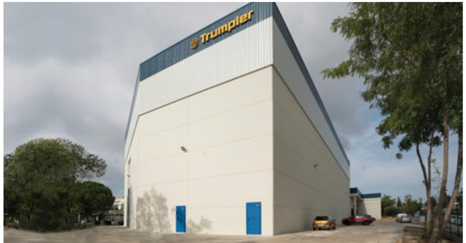
site's design was based on the dimensions of the automated warehouse to make full use of the available space, i.e., the racks were designed first and then the building was constructed. Thus, Trumpler obtained a 2,512 pallet storage capacity for raw materials and finished products.
